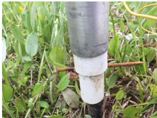
Installed Ground Mounting Assembly
