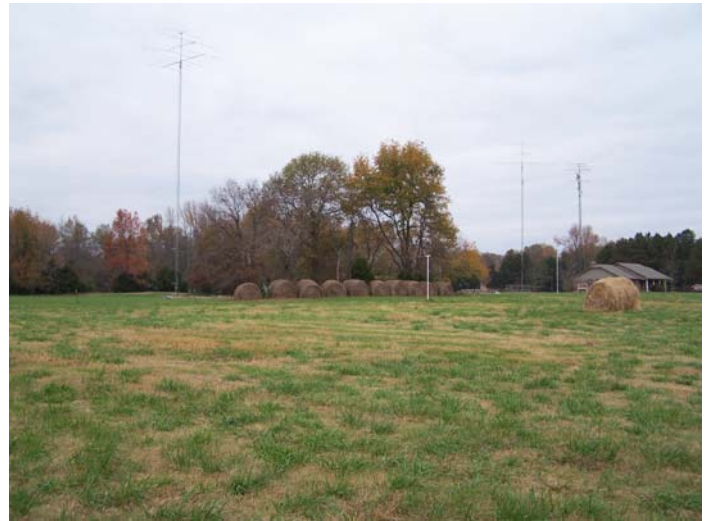
Figure 15 – 160 Meter Transmit Antenna (Left Tower)
