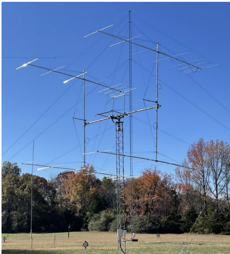
Figure 14: The completed 4x7 LFA 50 MHz EME array
