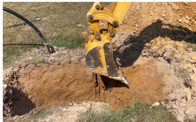
Figure 3: Old base hole is now ready for new Rohn 55 tower base
