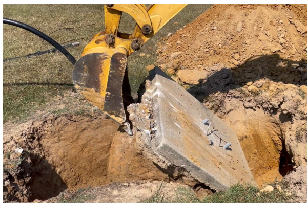
Figure 2: Old base is pulled into new hole
