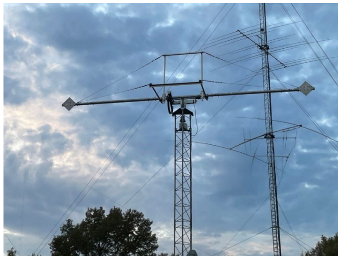
Figure 8: Installed H-frame without vertical booms
