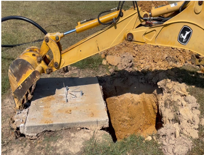
Figure 1: Hole dug to contain the old concrete base.
